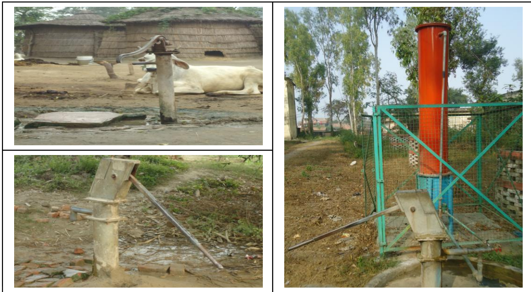
Different types of hand pump: Traditional hand pumps, India Mark hand pumps and the India Mark with special filters
