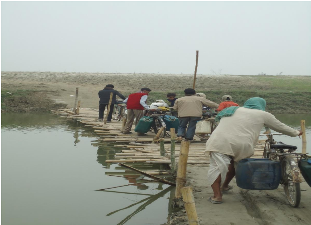
The bridge built by the local people with indigenous materials
