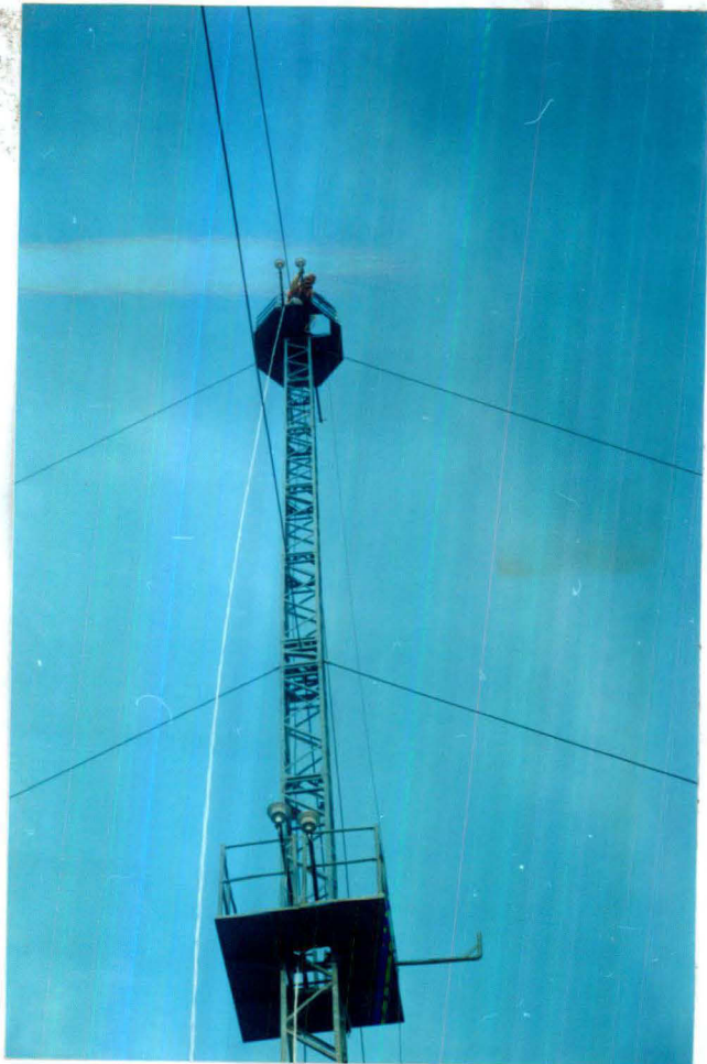
Figure 2.4 Photograph showing the installation of sensors on the 28m tower in progress. The temperature and humidity sensors are facing south-west while wind vel. & dir. sensors faces south-east
