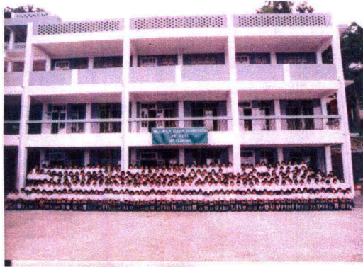
The new school building constructed, Pi Teii Building
