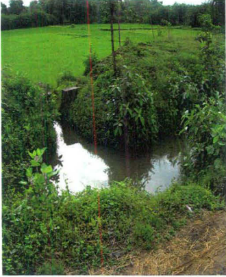
Channel desilted in Anthagudi
