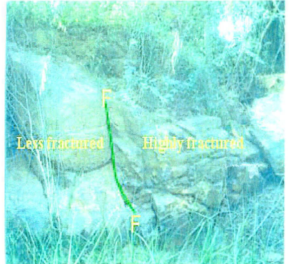
Two sets of fracture in ferrogenous quartzite along a microfault in RR Hospital
