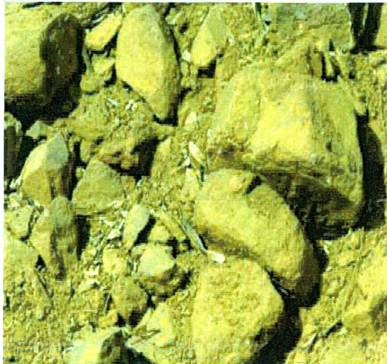
Fractured ferrogenous quartzite showing weathering and brittleness In JNU
