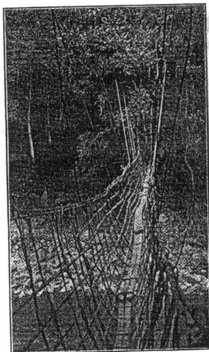
ANGAMI BRIDGE AT JESSAMI
