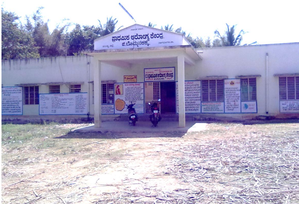
Health Sub- Centre at Soligarakopallu, G. Bommanahalli Gram Panchayat, Mandya
