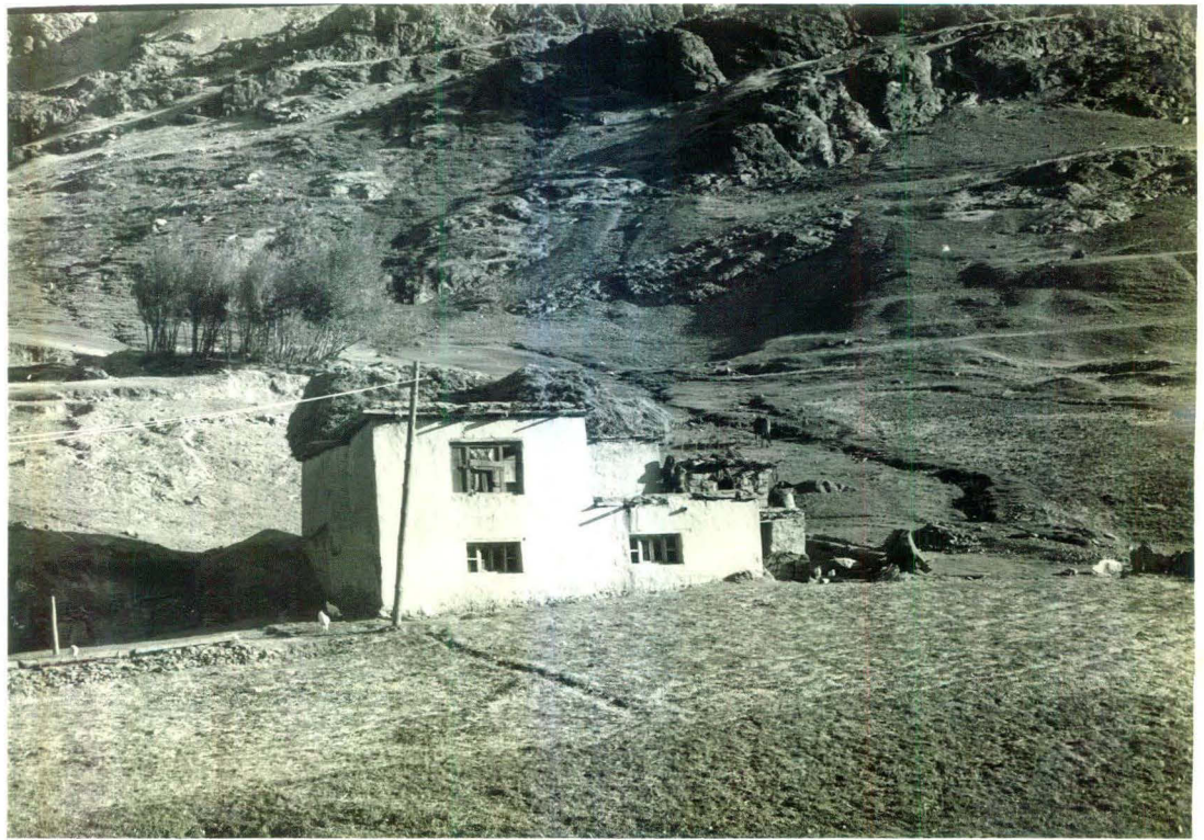
IV.6 A Typical Double storeyed House.
