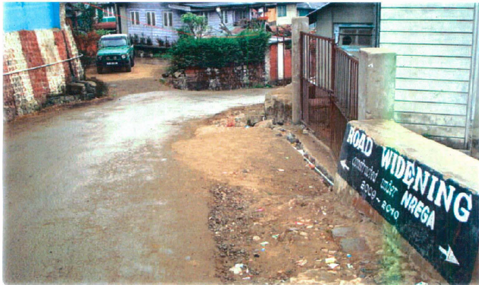
Figure 5 this picture shows a road widening constructed under NREGA project, 2009-2010.
