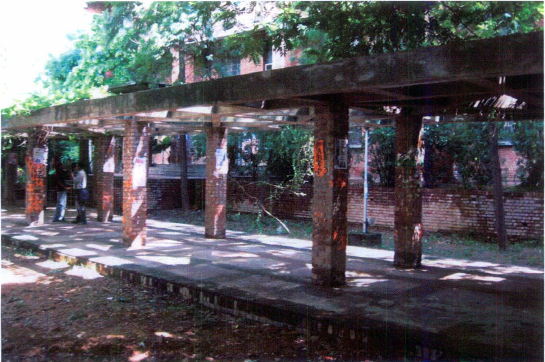
Fig. 42. Interconnecting Pathway/Terrace, School Building, JNU.
