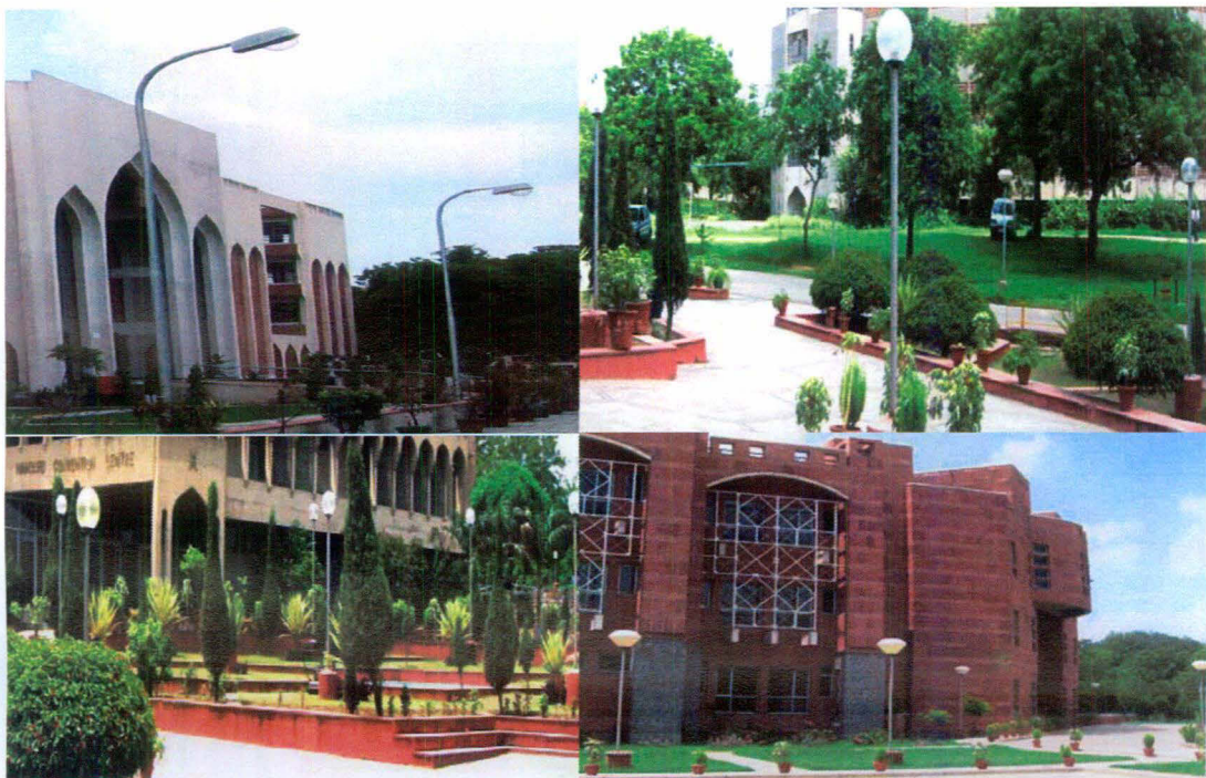
Fig. 28. Pictures shows the lighting system, Jamia Hamdard.
