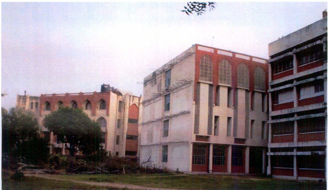
Fig.18. Annexure Buildings, Faculty of Unani Medicine, Jamia Hamdard.
