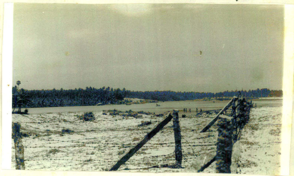
Plate.6. Fenced cultivation of Acacia and Eucalyptus. Failed attempts at estuary stabilization
