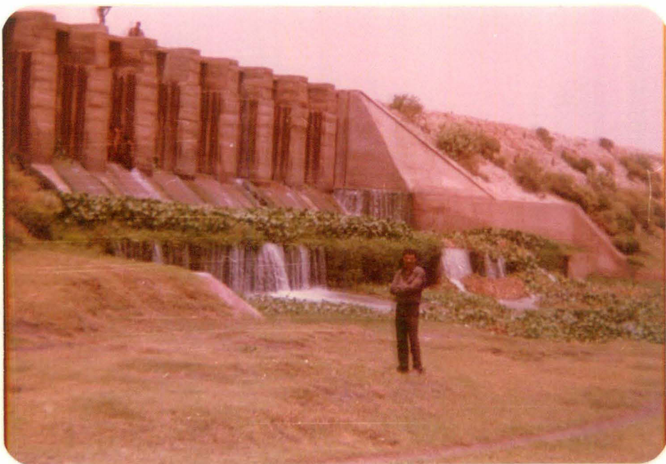
STATION NO. 4 OF ASH POND.
