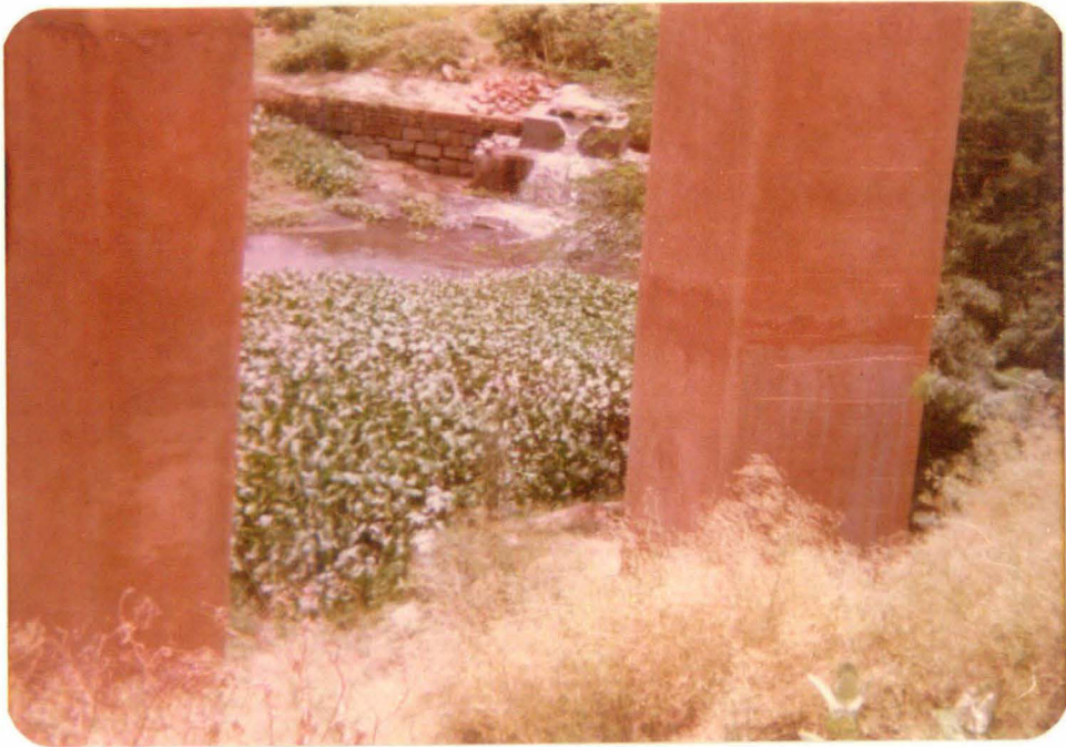
STATION NO. 3 OF PARTIALLY TREATED SEWAGE
