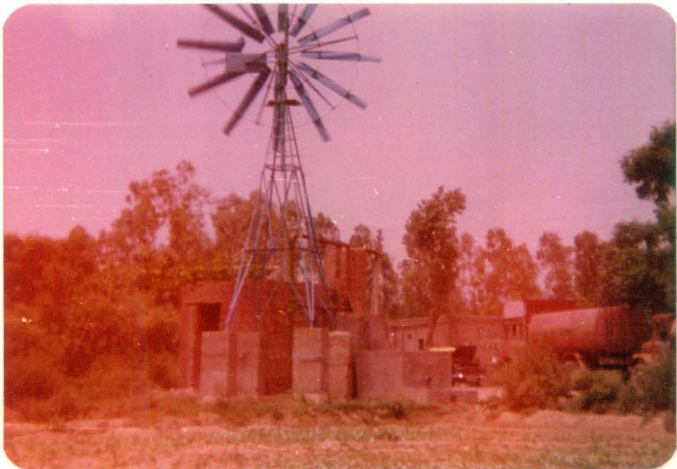
STATION NO. 20 OF GROUND WATER (OPEN DUG WELL FITTED WITH WINDMILL)
