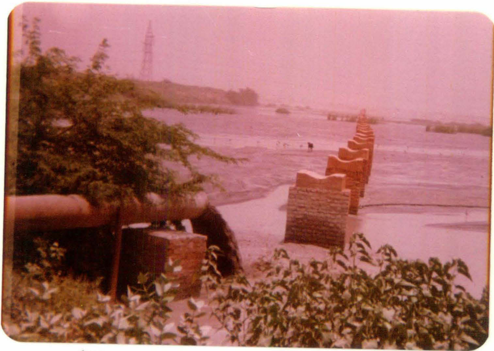
STATION NO. 1 OF ASH POND.
