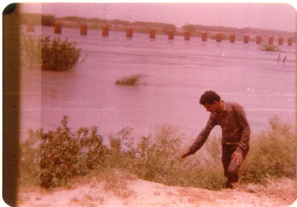
STATION NO 2 OF ASH POND.
