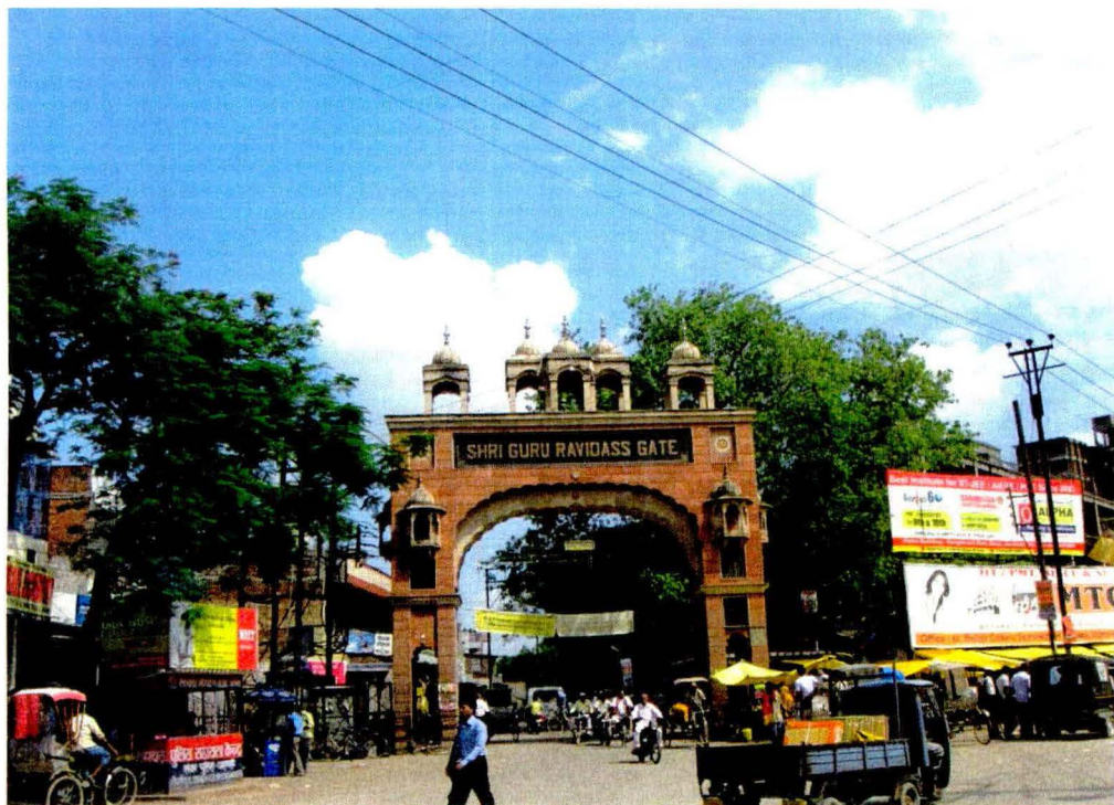
Figure 09: After completion of the gate.
