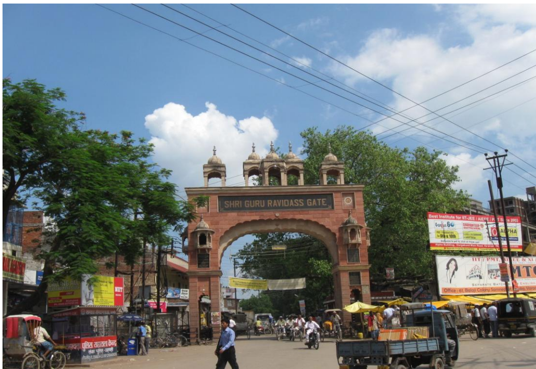
Figure 09: After completion of the gate.
