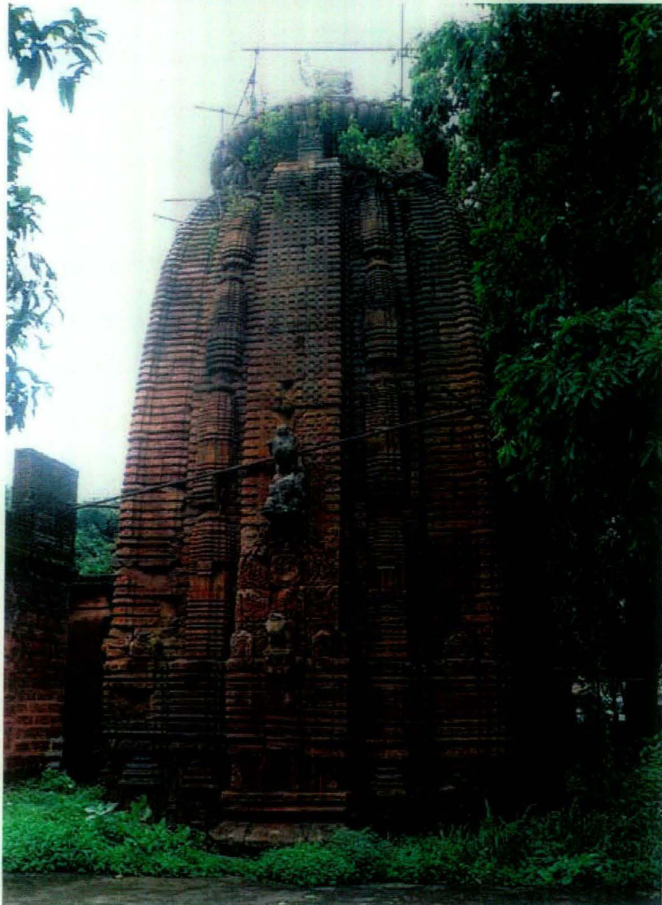
Fig.24. Amūnhā Deūla, General View
