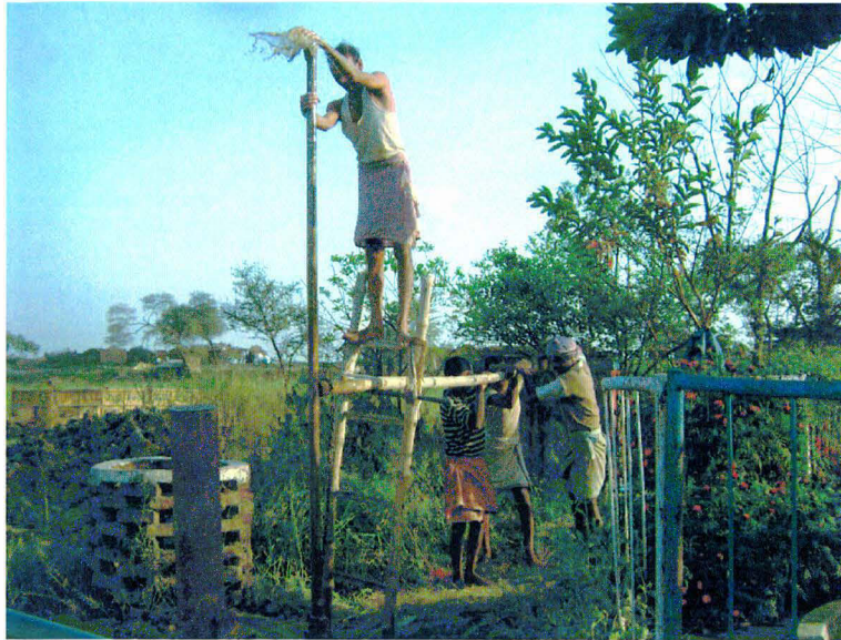
1. Drilling in progress
