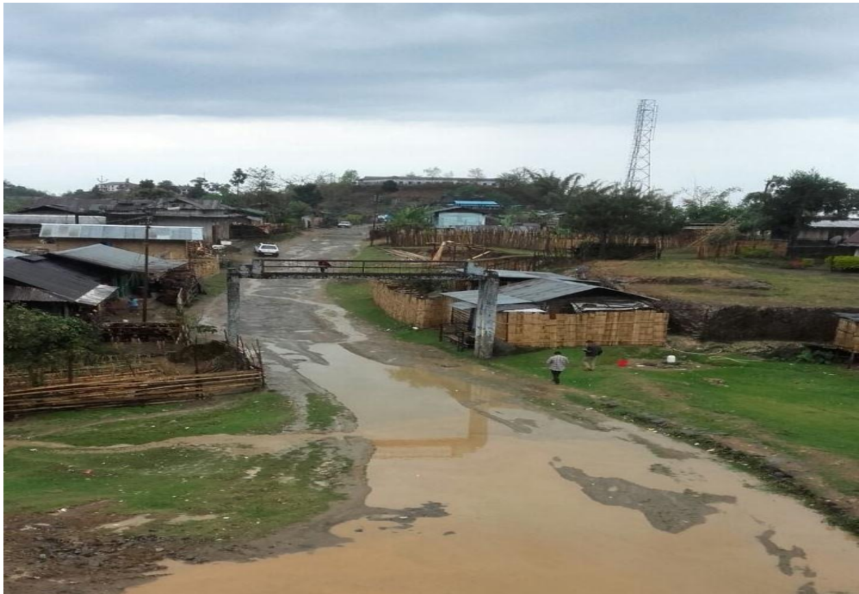
Image 3.7: Picture showing the poor condition of the road at the entrance of the town
