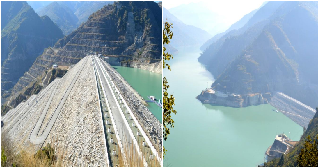
The colossal structure of the Tehri dam at 260 m. Photo taken from the top of the dam (2.12.14), as the road from the dam swirls down. The 60 km long lake behind it has inundated the best agricultural land along the banks of the river Bhagirathi, and is leading to the ceding of close to 30-40 villages.
