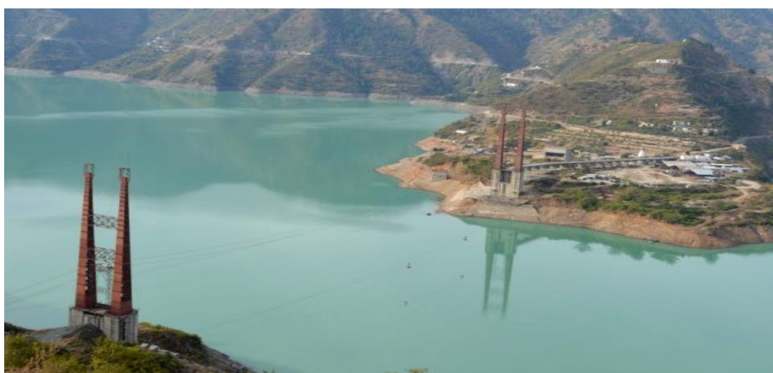
Dobra Chanthi bridge, that is said to be lifeline for people who have been marroned on either side after formation of Tehri lake, has become a symbol of corruption (19.12.14).
