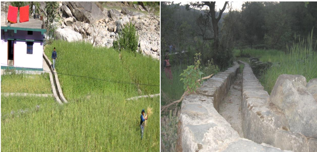
Dry Kuhls Photos taken on 24.3.2012 in Rudraprayag, first shows the how the Kuhl water is used for irrigation in the Augustmuni town, second photo is of a kuhl running dry in Rayadi village. Most Kuhls are running dry now as the rivers have been diverted or choked due to muck dumped in rivers by hydropower projects.
