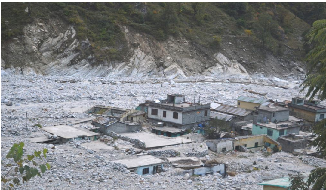
The village Pulna under debris in the Bhyundar ganga valley in Chamoli. A 24 MW project near the village (within 10 Km from the protected area of Valley of Flowers) was under construction (Photo 4.11. 2015)
