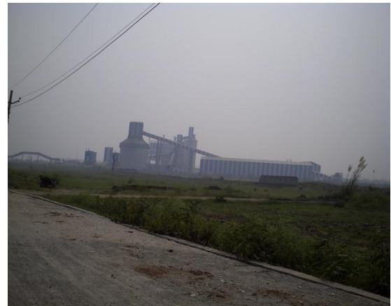
Example of industrial development in the village
