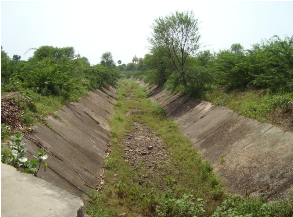
Figure 6.6: Canal passing through Jaisamand dam
