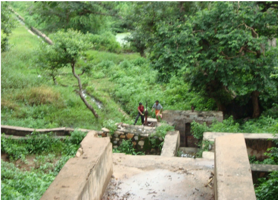
Figure 6.2: Canals passing through Siliserh dam
