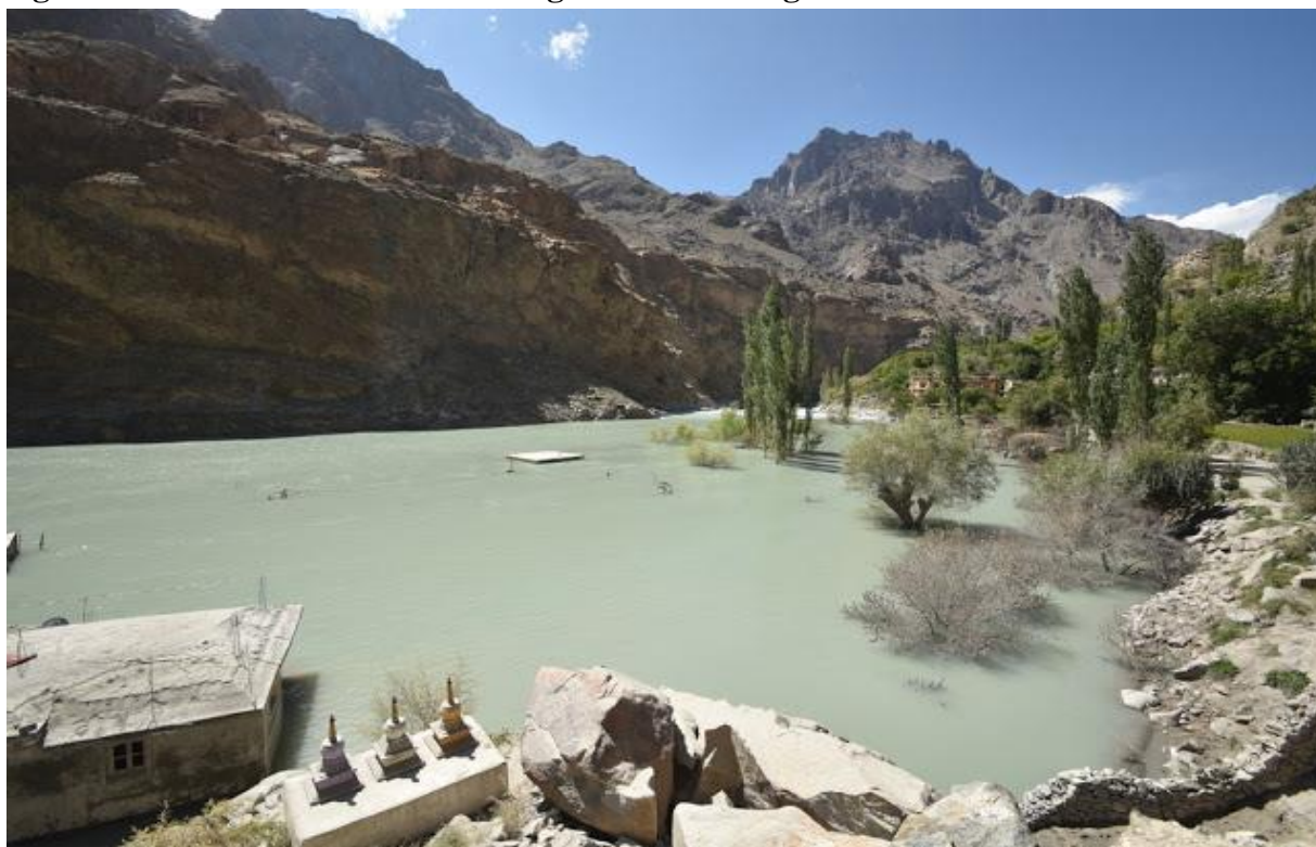
Figure 7:View of Indus River Blockage in Bema village.
