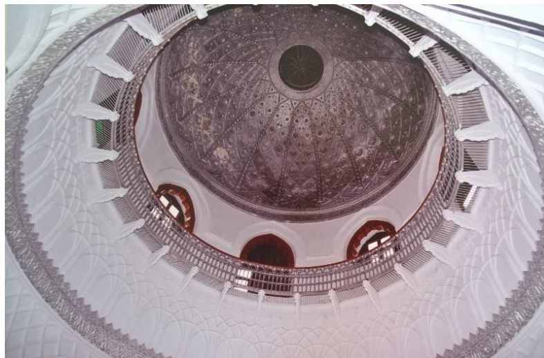
Image 73: Dome above the Octagonal Lobby Source: Souvenir Committee, High Court, Madras (2012)
