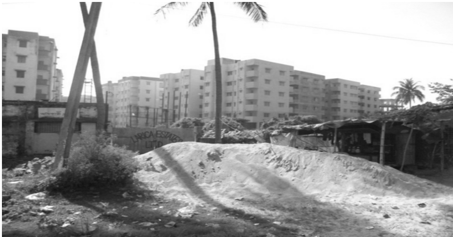
Figure 3: Larica estate township project beside Barrackpore Road 2 (source: author)
