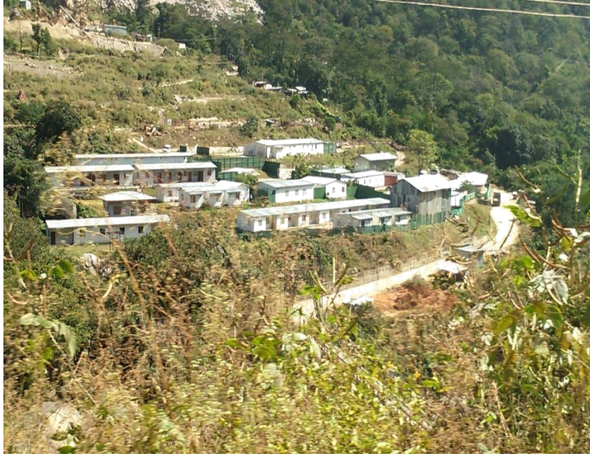
Picture 18: Agricultural lands cleared for the construction of quarters and offices.
