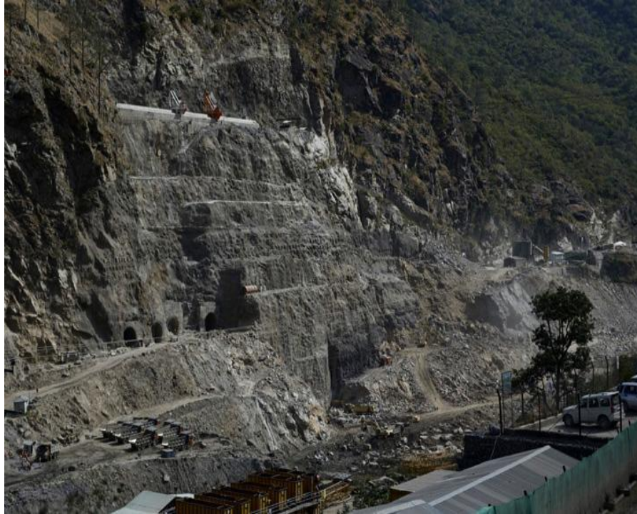
Picture 14: Punatsangchu- I Dam construction 7
