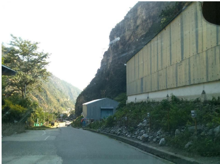
Picture 17: Temporary sheds made of corrugated sheets in the roadside of the Punatsangchhu project area
