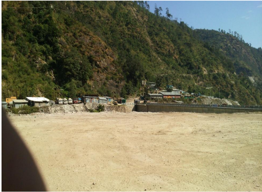
Picture 8: Dumping sites in the Punatsangchhu Project
