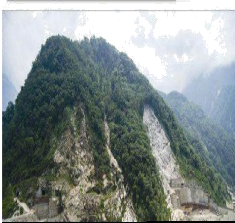
Picture 31: Landslide in Dzongu in August 13, 2016
