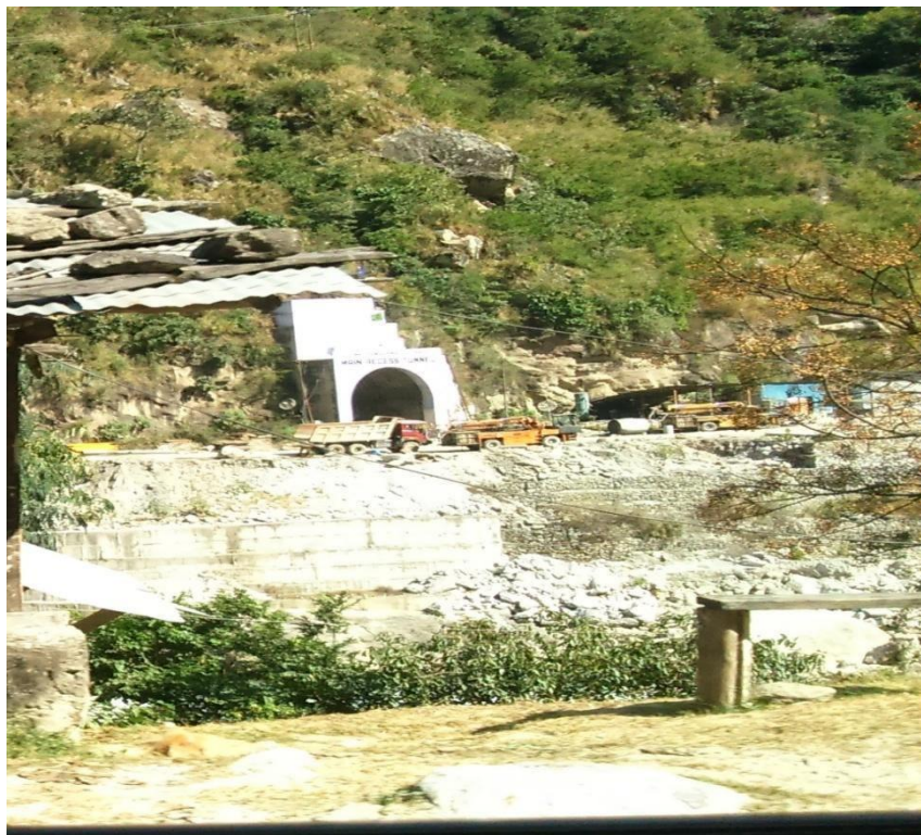
Picture 13: Tunnel of Punatsangchhu- I project
