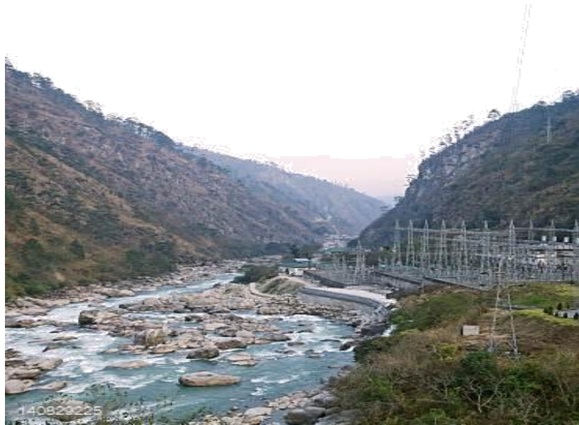
Picture 16: Punatsangchhu Project Construction site 8
