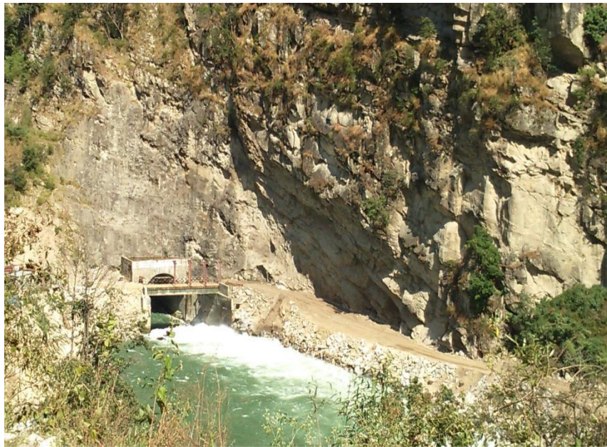
Picture 11: Water outlet tunnel Punatsangchhu-I project
