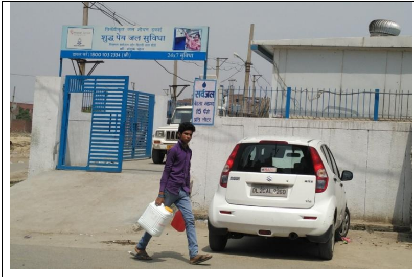
Photo 6.3: The Main Sarvajal Plant at Savda Ghevra
