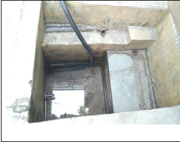
Photo 5.2: Trench in Nehru Ekta Camp for Collecting Water (DJB Managed Area)
