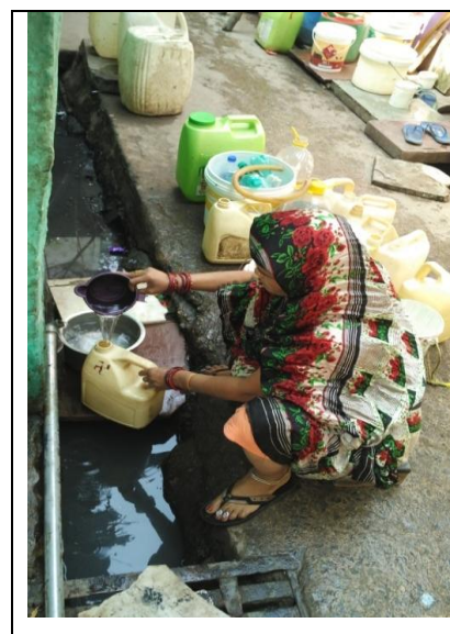
Photo 5.1: Position of Water Supply Pipeline in Karotiya Camp
