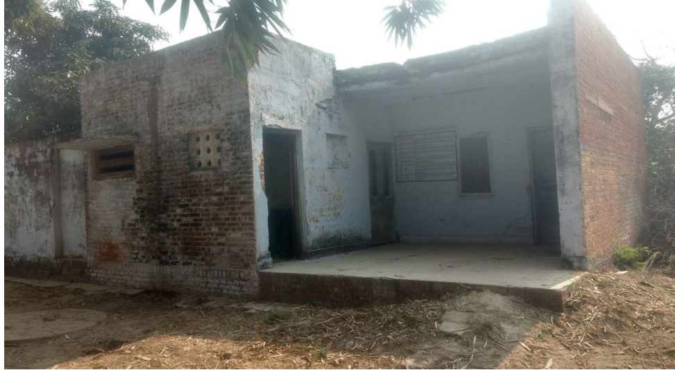
Sub-Centre of the Majhwara Village, Sultanpur
