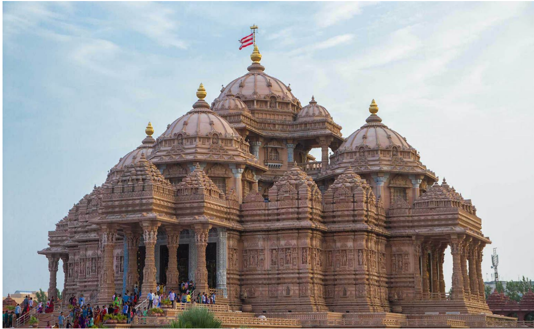
Figure 5.1: Akshardham (by BAPS, http://akshardham.com/download/photo-galleries/moods-of-akshardham/#&gid=1&pid=11 ).
