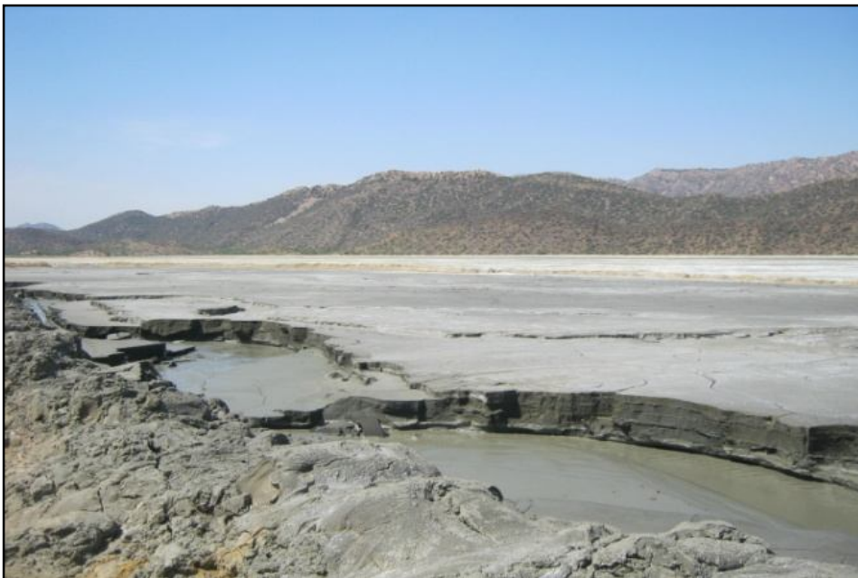
Fig. 2.5 Tailing dam at Khetri
