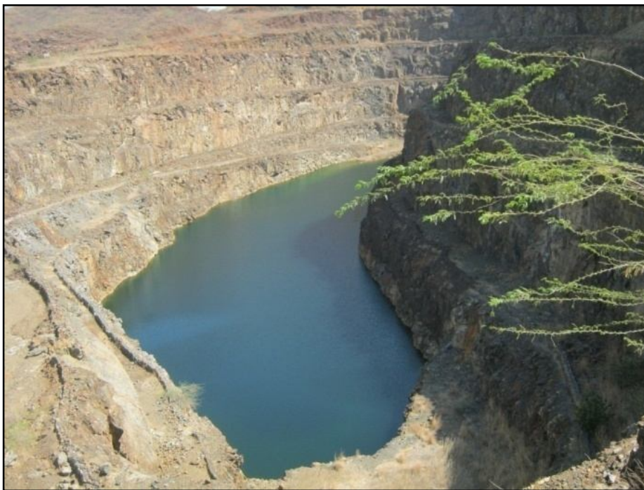
Fig. 2.6 Abandoned Chaandmari mine with acidic water (pH~ 4)
