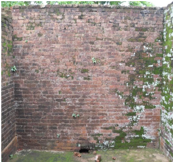
Figure 3.9. One of the walls of the cells in Monastery I
