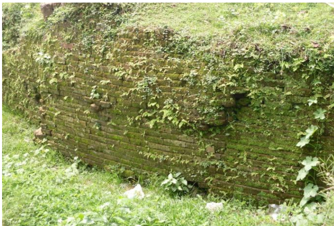
Figure 3.5. Sections of the trenches showing the brick structures buried beneath the mound.
