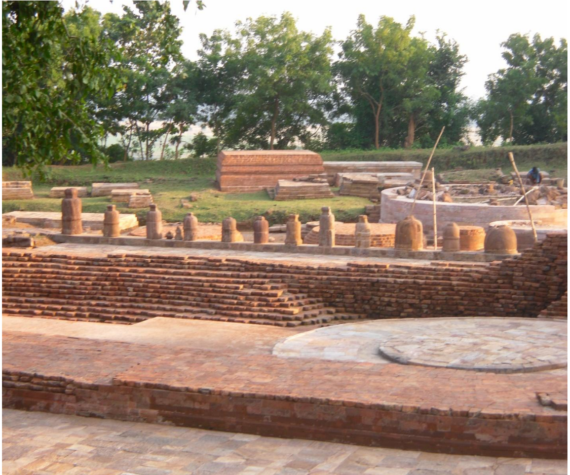
Figure 3.13. The Chaityagriha area undergoing restoration work, Lalitgiri.
