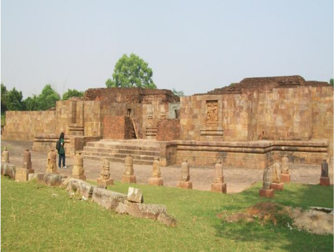
Figure 2.4. The side view of Monastery
