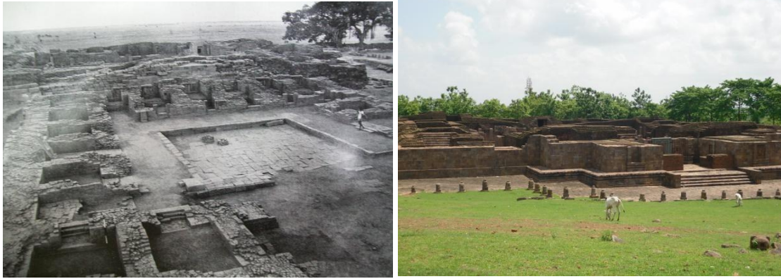
(Left) Figure 3.10. The area of Monastery I during excavation, (Mitra 1981: Plate cxxvi); (Right) Figure 3.11. Monastery I
